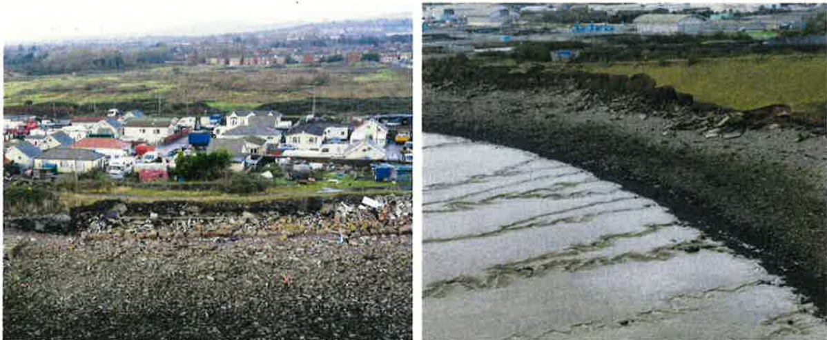
Figure 3: Existing coastal defences to the west of the mouth of the River Rhymney
